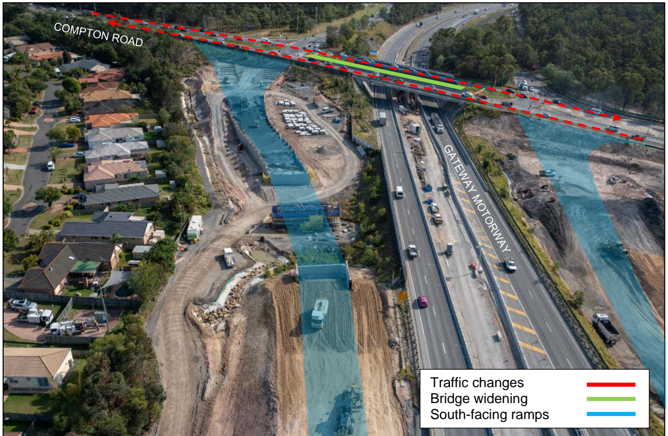
Above: Gateway Motorway / Compton Road interchange looking north, September 2018
