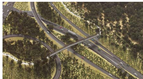
Image above: Artists' impression of the pedestrian and bicycle overpass at Mt Lindesay Highway/Beaudesert Road interchange, to be built as part of the Logan Enhancement Project.
